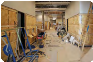
Sound-absorbing material (under construction)
